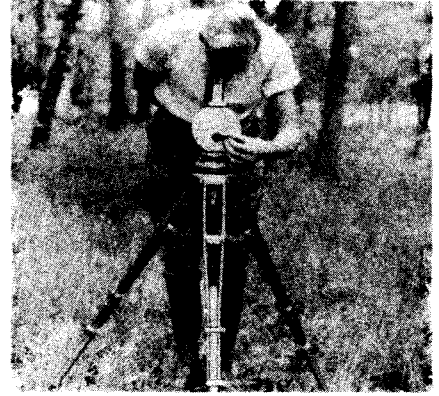
Field balances for magnetic surveying.
